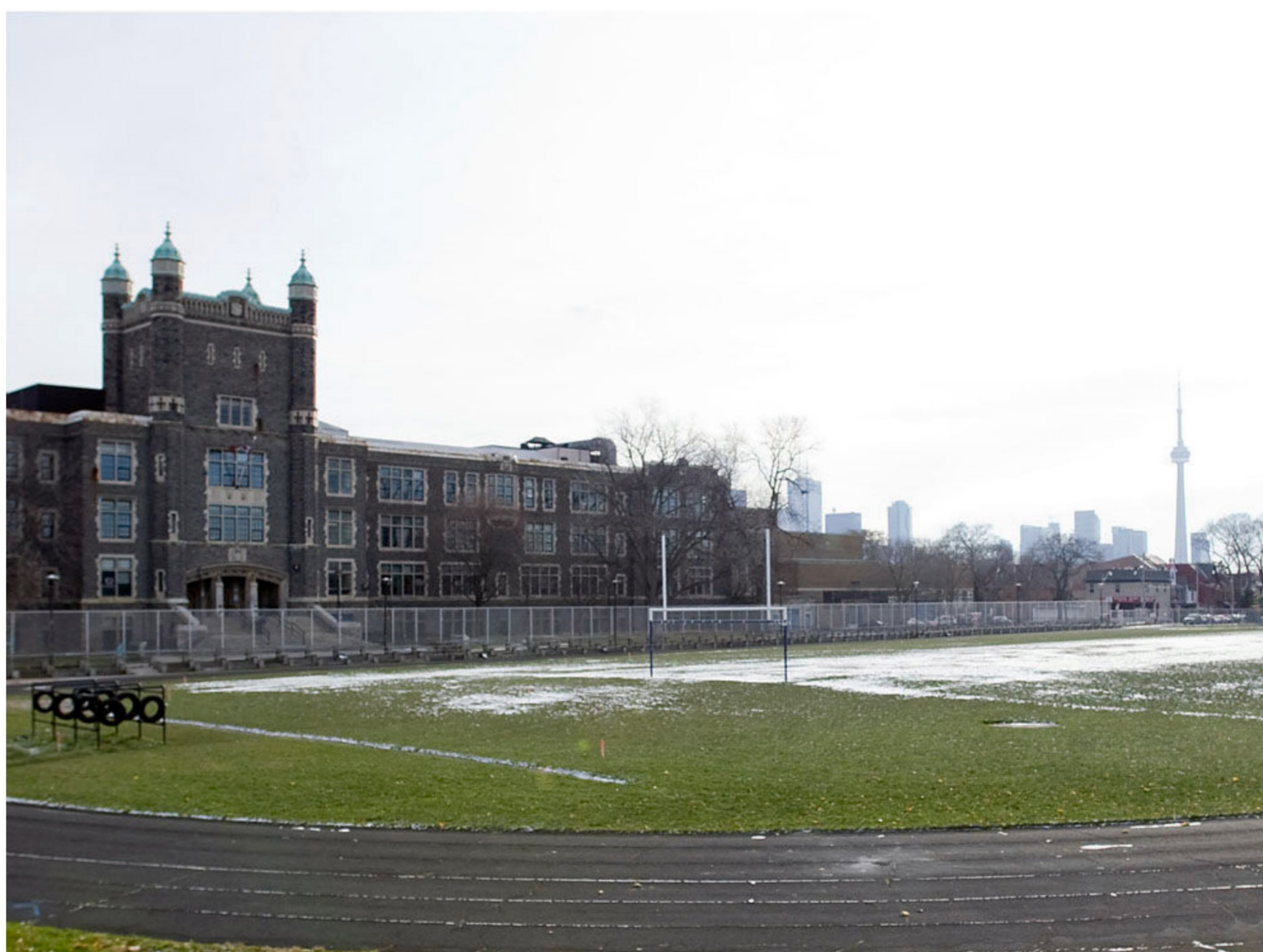
The field at Central Technical School is being considered for a winter dome, which has residents in the area coming divided. - Photo/STAFF
